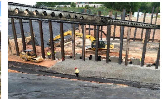
Installation of the MSE Wall at Bridge Abutment
