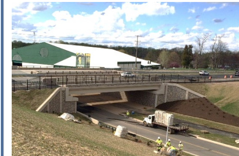
Dual single-span bridges along Route 123
