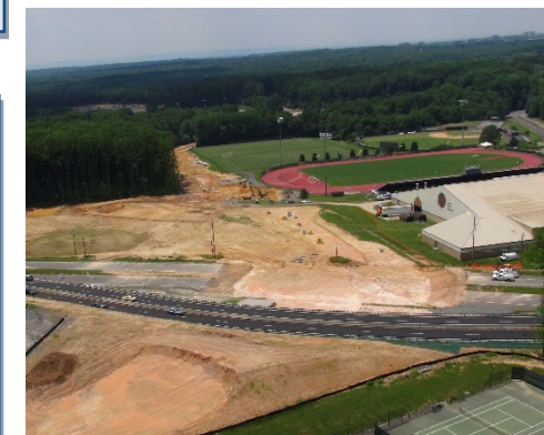
Grading for new location roadway
