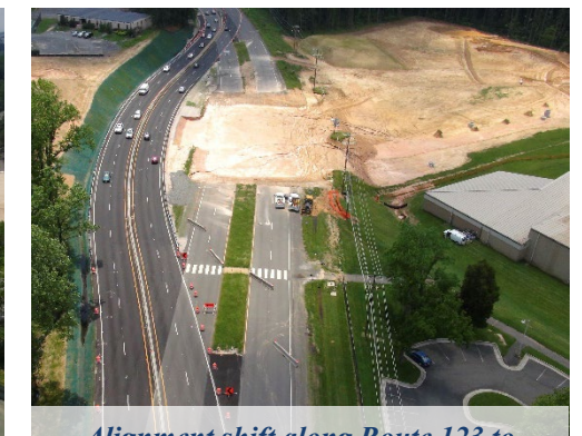
Alignment shift along Route 123 to allow for bridge construction
